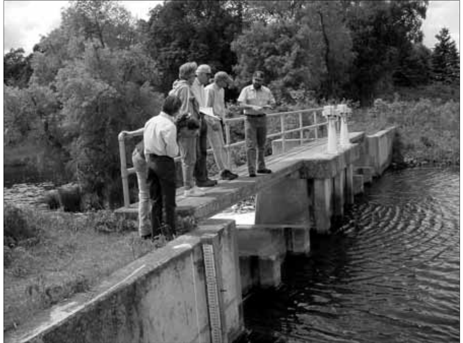
Lowell Deede discusses water control at the Chippewa Lake structure.
